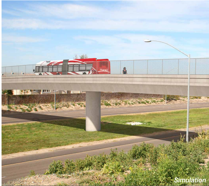
Transit guideway bridge over South Bay Expressway
