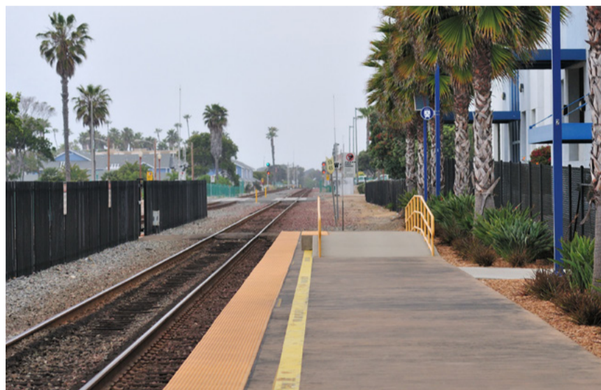
Crews will be working to extend the easternmost COASTER/Amtrak platform.
