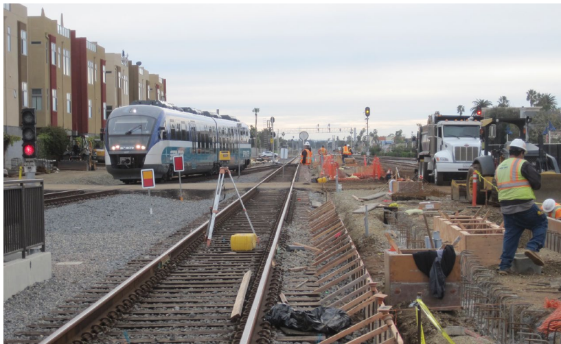
Crews work on the new platform at Oceanside Transit Center
