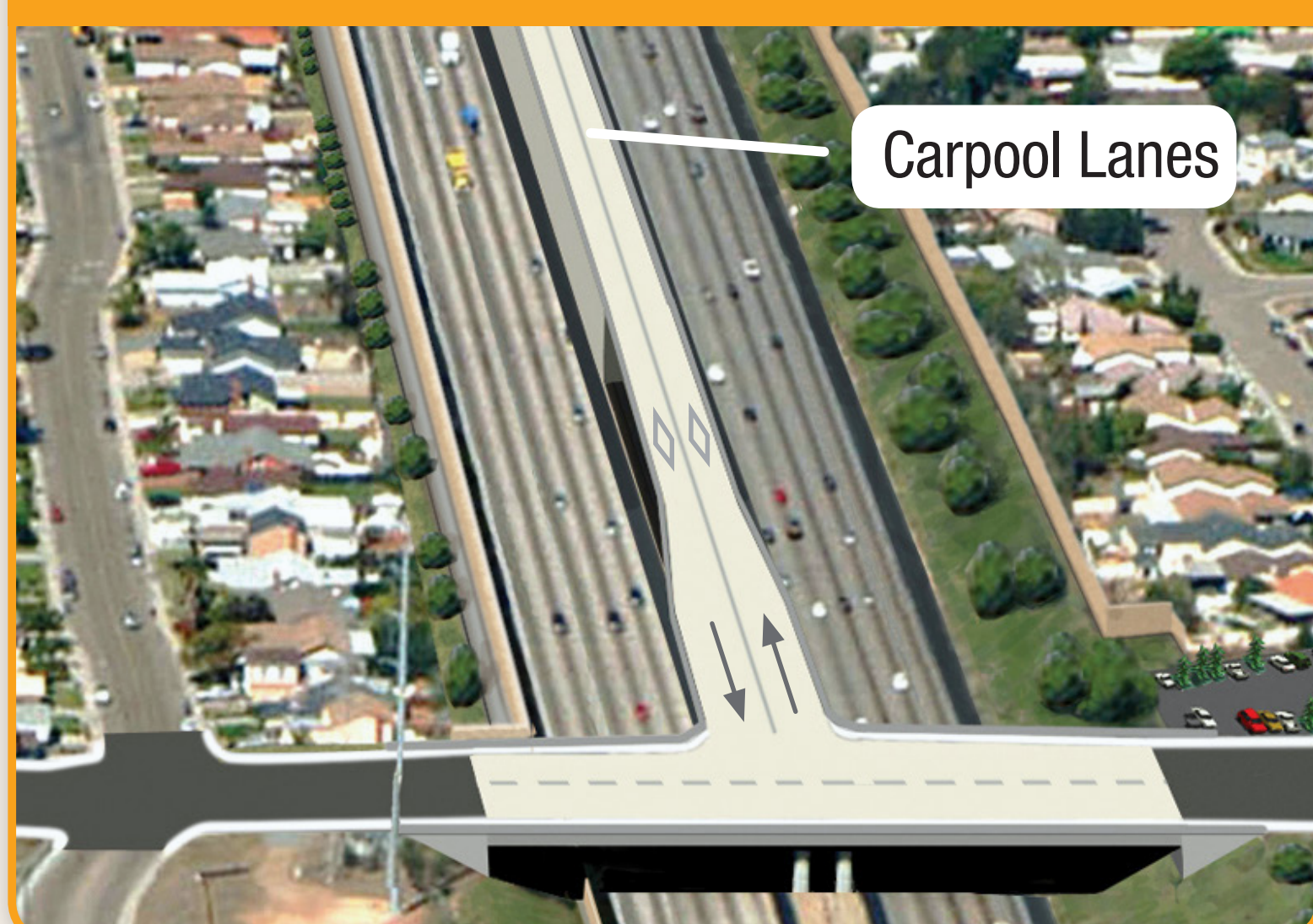
Direct Access Ramps connect the carpool lanes to local surface streets.
