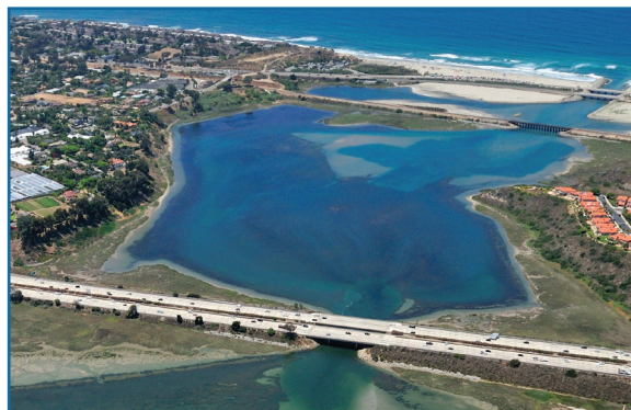
Batiquitos Lagoon (shown above), along with San Elijo and Buena Vista lagoons, will include longer bridges for improved tidal flows.
