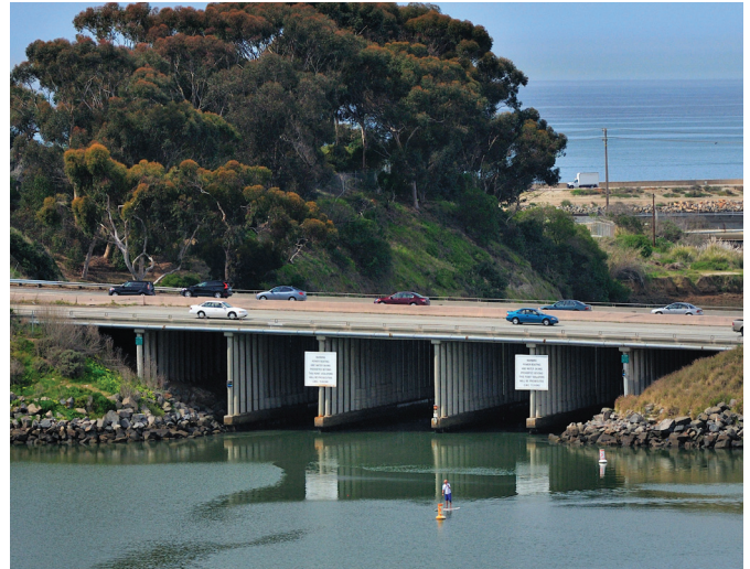
The I-5 NCC Project includes replacement of the Aqua Hedionda bridge to reduce the number of columns in the lagoon.
