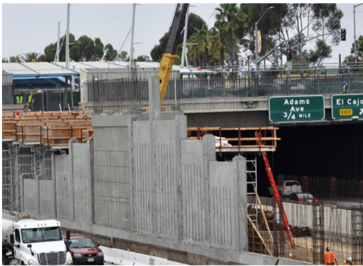
Crews continue to build the pedestrian bridge south of University Avenue.
