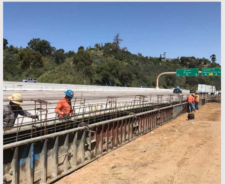
Construction crews set rebar for the northern section of the concrete barrier that will separate the SR 15 Commuter Bikeway from the freeway. This northbound view is approaching the project's endpoint at Camino del Rio South.
