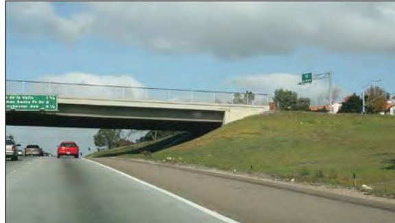
An example of a short seat abutment.
