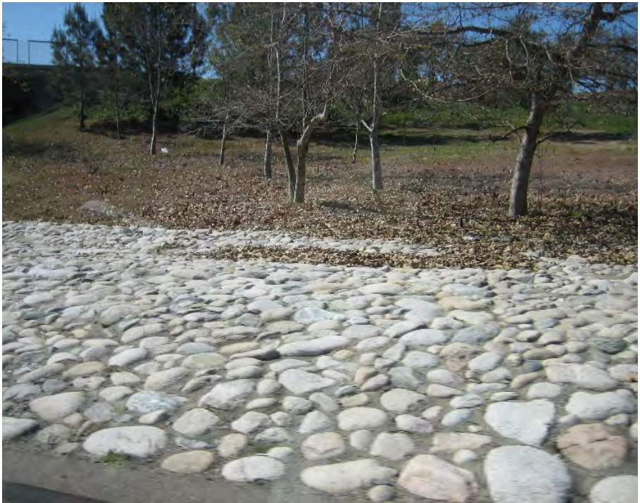
Rounded creek cobble could be used where possible for slope paving under the bridge structures and in areas of the project that are too shady to plant
