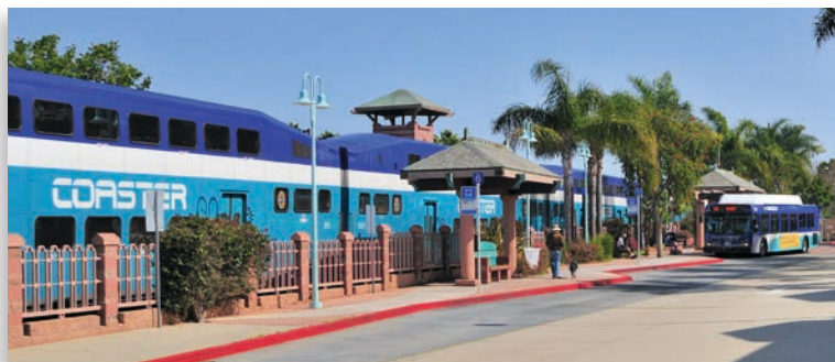
The project will add 1.1 miles of second main railroad track from southern Oceanside to Carlsbad Village
