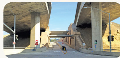
Existing north-facing Direct Access Ramp
