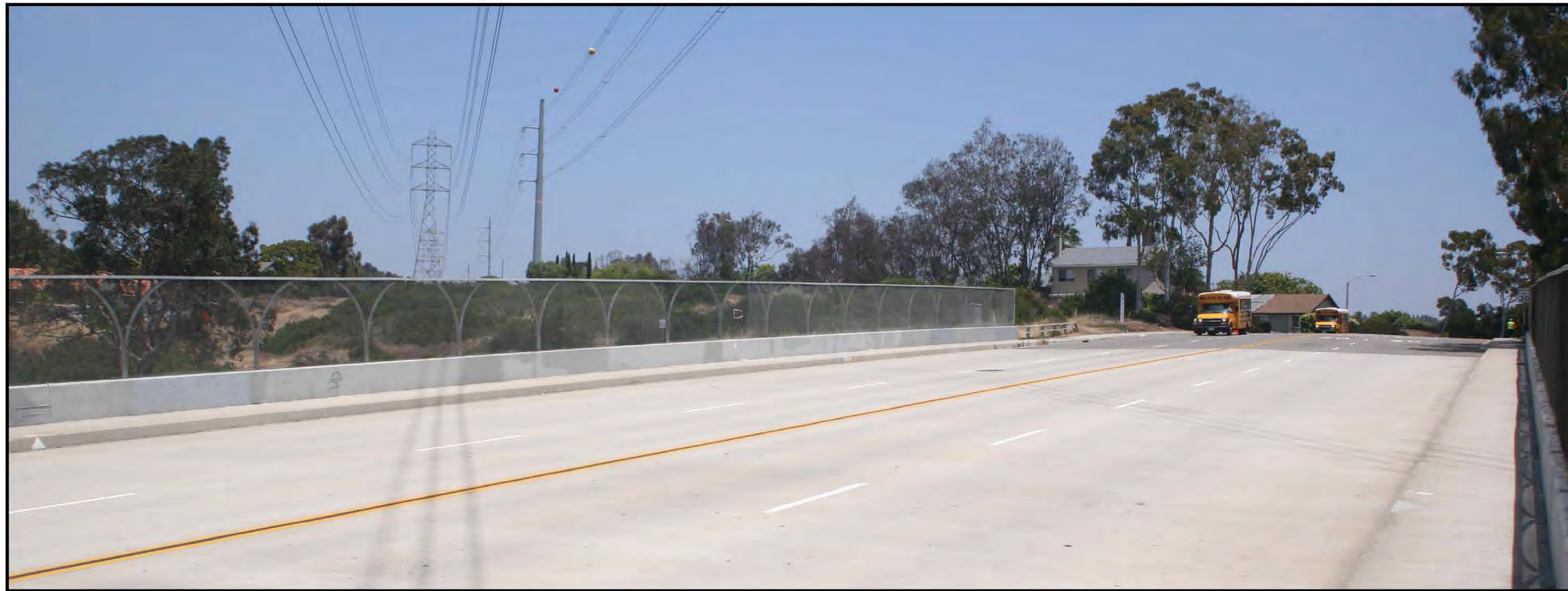
Existing View - Looking Northeast from the East Palomar Street Bridge
