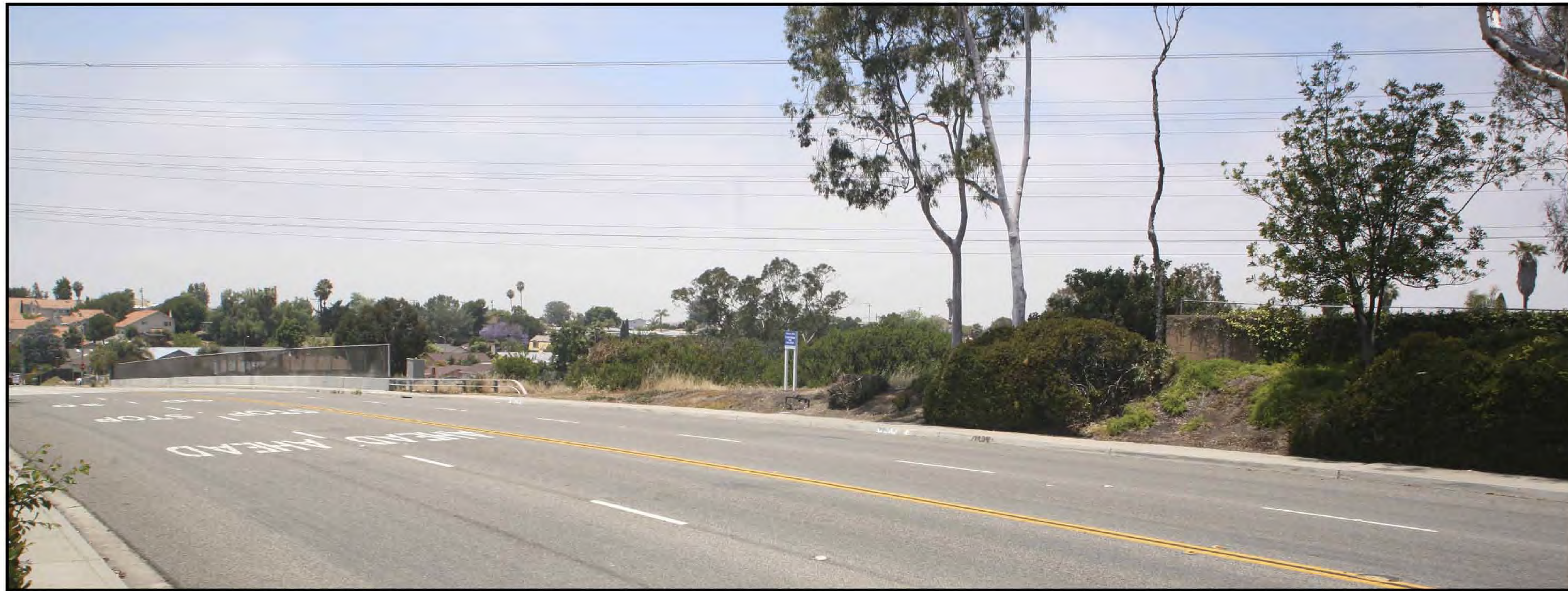
Existing View - Looking West at the East Palomar Street Bridge
