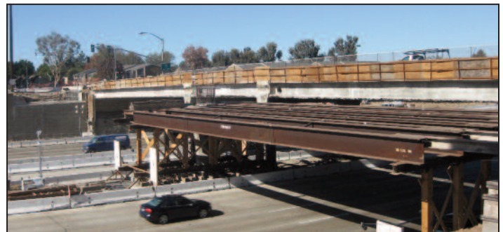
Temporary bridge support beams over I-15 at Carroll Canyon Road.
